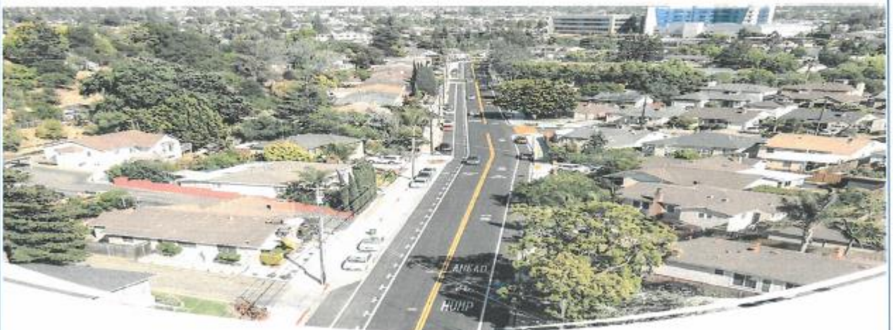
Stanton Avenue Sidewalk Project
